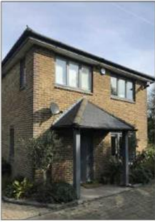
Front elevation and entrance porch
